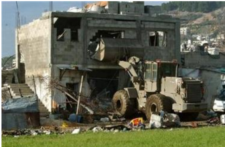
Construction projects (demolition)
